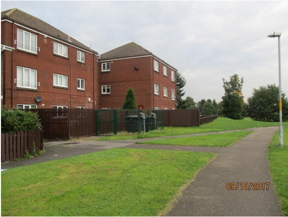
Three storey building at the end of Lyneham Close
